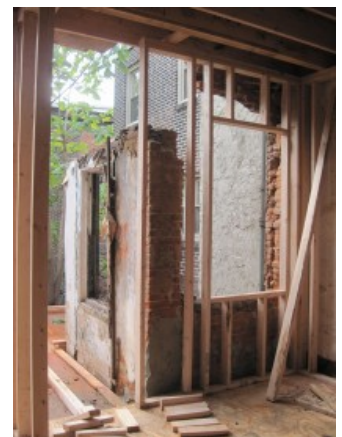
Framing for one of the apartments on the second floor.
